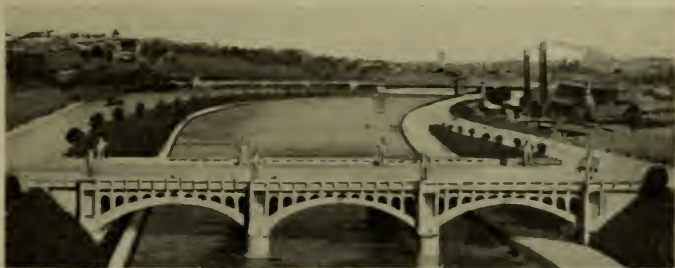
PROPOSED REINFORCED CONCRETE BRIDGE AT YARRA.
